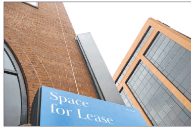
Office space is available for lease in the Plaza of the Rockies complex on South Tejon Street in downtown Colorado Springs.
