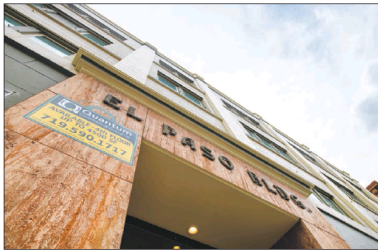
A sign advertises office space that's available for lease on the fourth floor of the El Paso Building on Tejon Street in downtown Colorado Springs.
